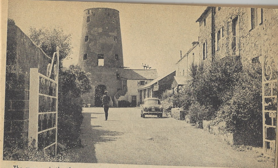
The museum is the three-story building on right of approach to Witches' Mill.
